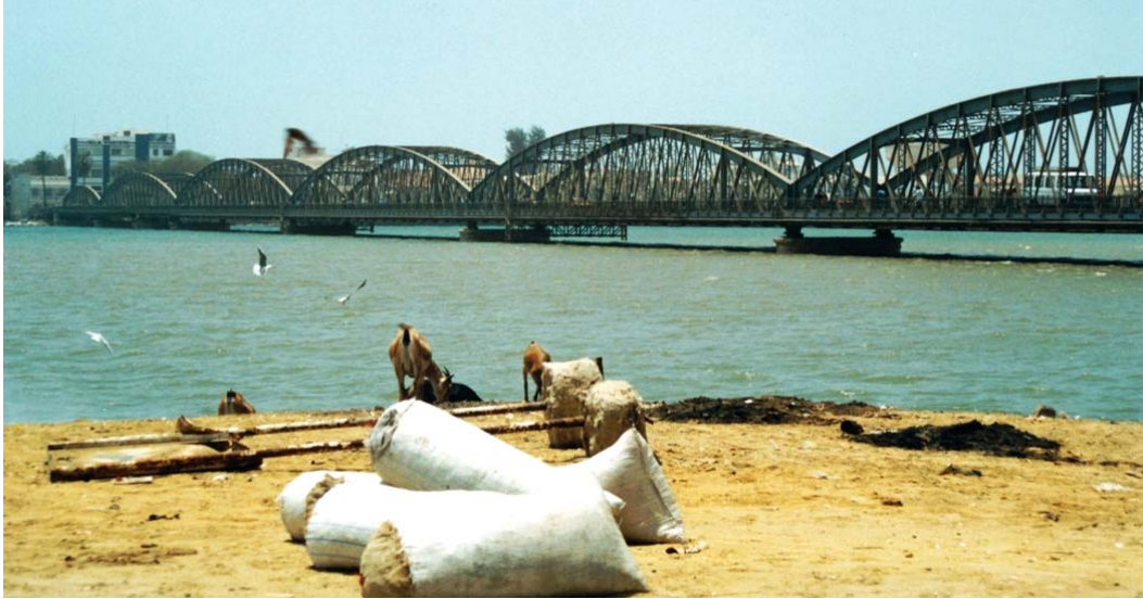
Above: The Faidherbe Bridge in Saint-Louis has 8 spans with a total length of 1600 feet (500 m).
